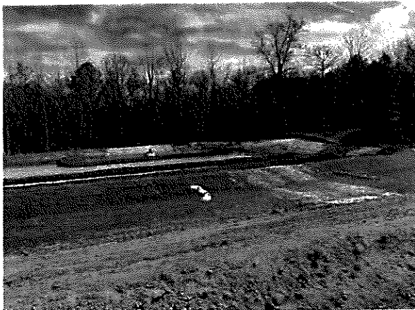
East facing - Detention ponds in good condition.
