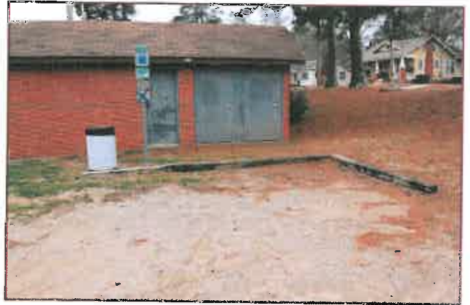
Existing Restroom / Concession Building
