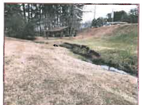
Daylighted Stormwater Channel
