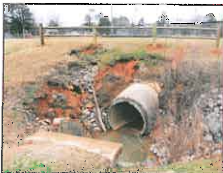
Daylighted Storm Pipe and Erosion
